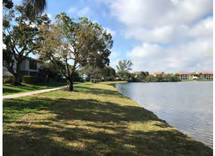
Figure 33: After Landshore's installation of Flexamat®
