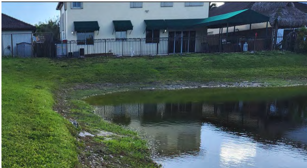
Figure 17: Bank Erosion with soil been lost and steep slope
