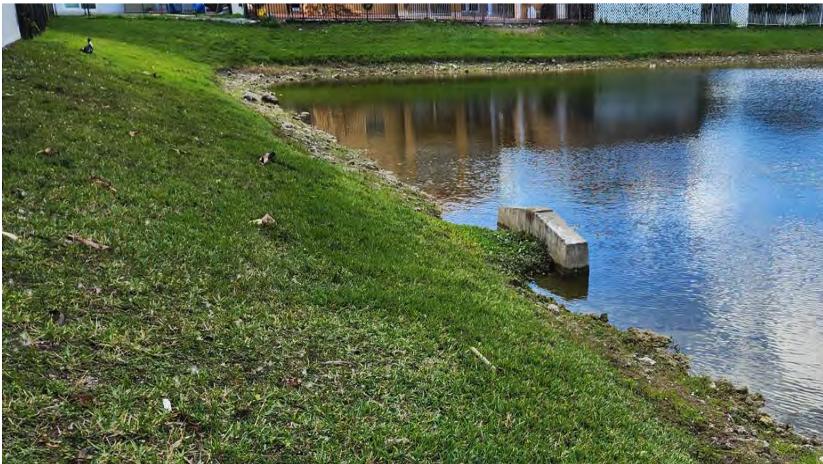
Figure 25: Bank Erosion showing loss of material and headwall is a good indication of where the soil supposed to be at.
