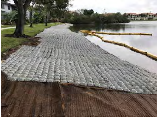
Figure 32: During Landshore's installation of Flexamat®
