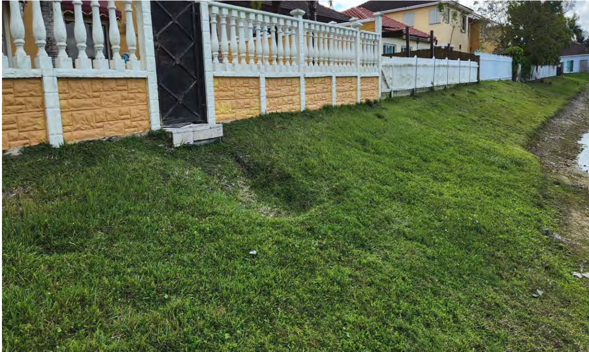
Figure 24: Bank Erosion getting closer to structures
