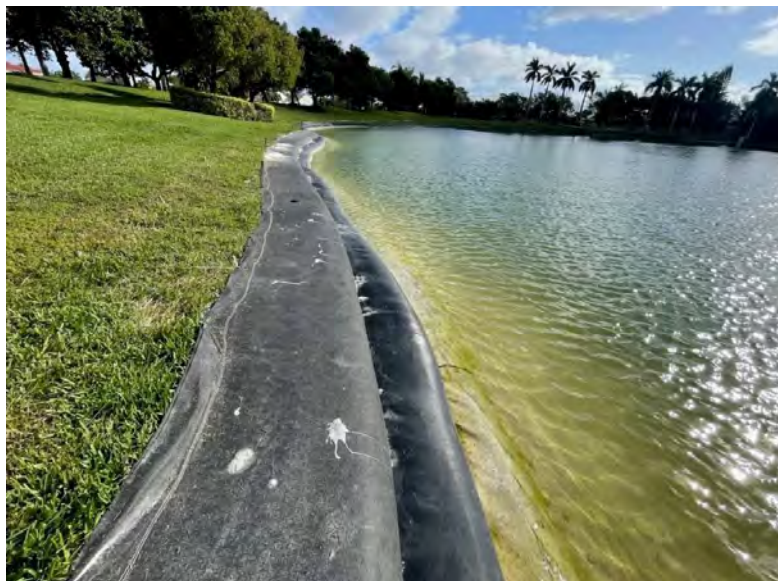
Figure 29: Example of EFT® Landshore's Installation
