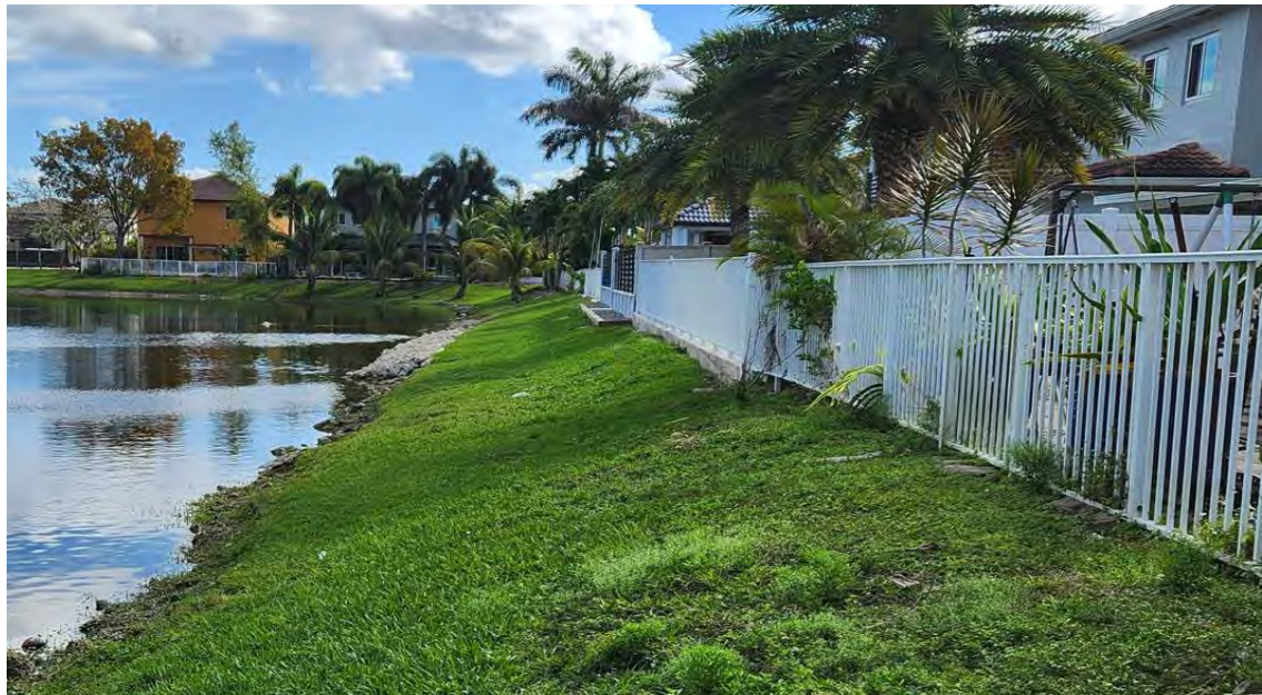
Figure 21: Bank erosion with uneven shoreline at water's edge
