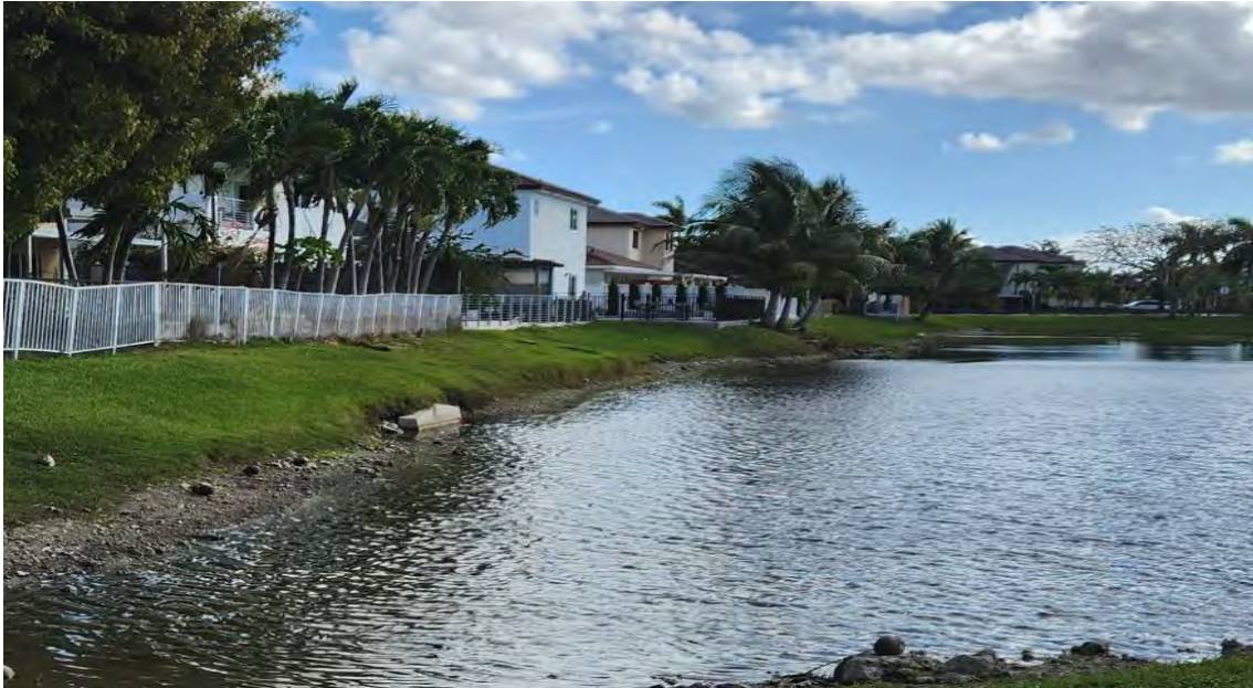
Figure 20: Bank erosion with steep drop off at the embankment
